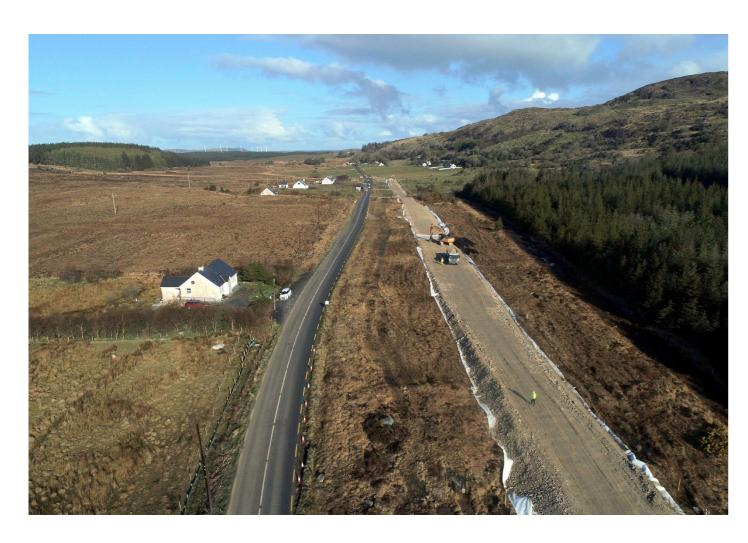
In January 2021, construction began on the N56 Letterilly to Kilraine Road scheme in Co. Donegal. The project comprises 4.1km of Type 3 single carriageway. ROD has been engaged by Donegal County Council to provide construction and handover stage consulting engineering services for the scheme, for which Wills Bros Ltd. has been appointed as the main contractor.
