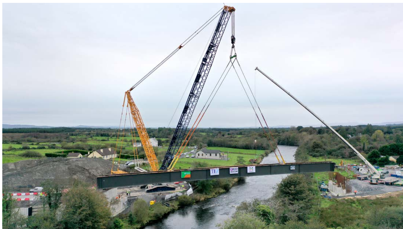
Cloongullane beam lift
