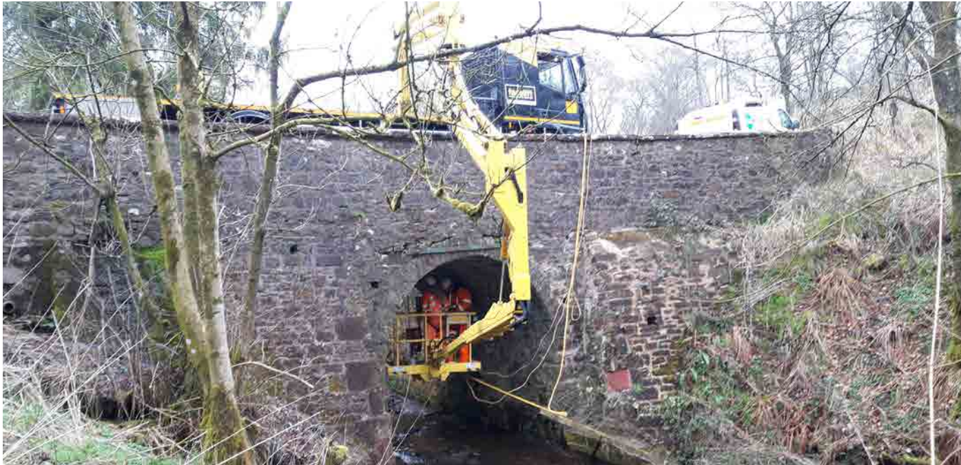
Underbridge unit in use during inspection of Holywell Bridge, Cumbria.
