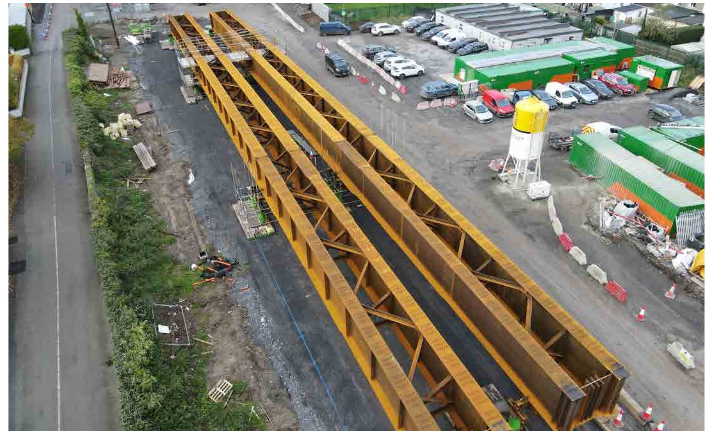
80m long braced steel plates girders.
