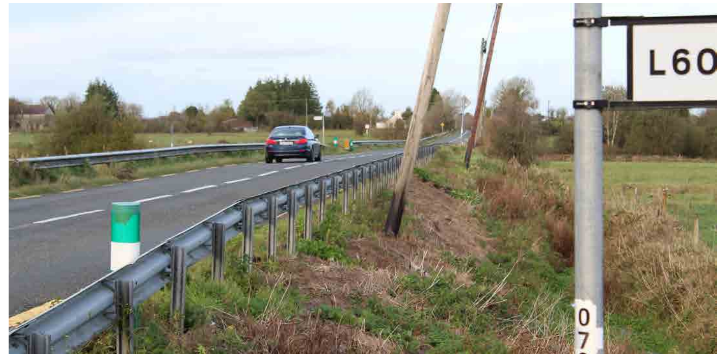
Site photo showing telegraph poles leaning due to poor ground conditions.
