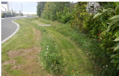
Typical urban swale detail.
