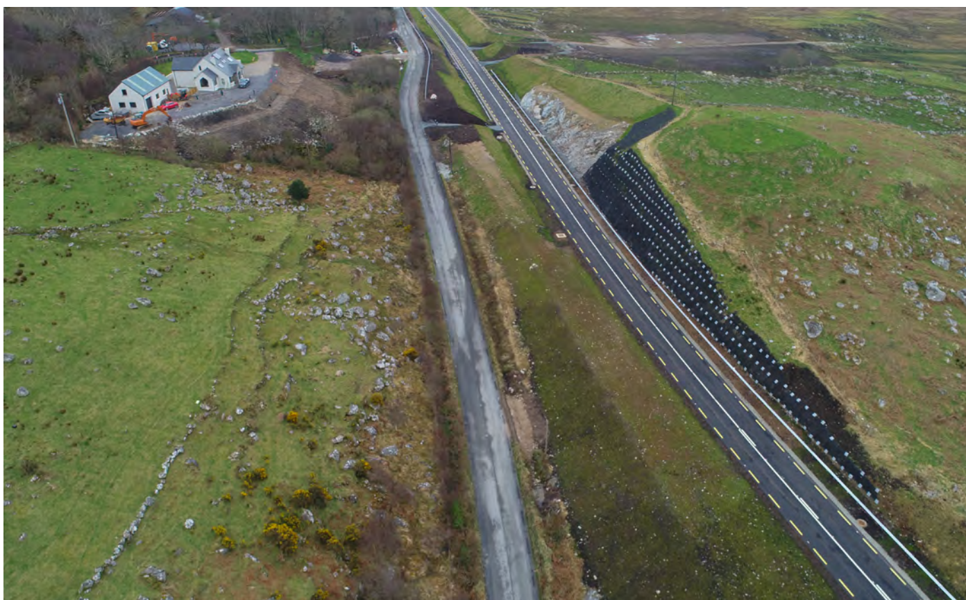
Aerial photograph of N56 Letterilly to Kilraine Phase 1, soil-nailing and rock excavations were needed for steepened slopes avoiding a national monument.
