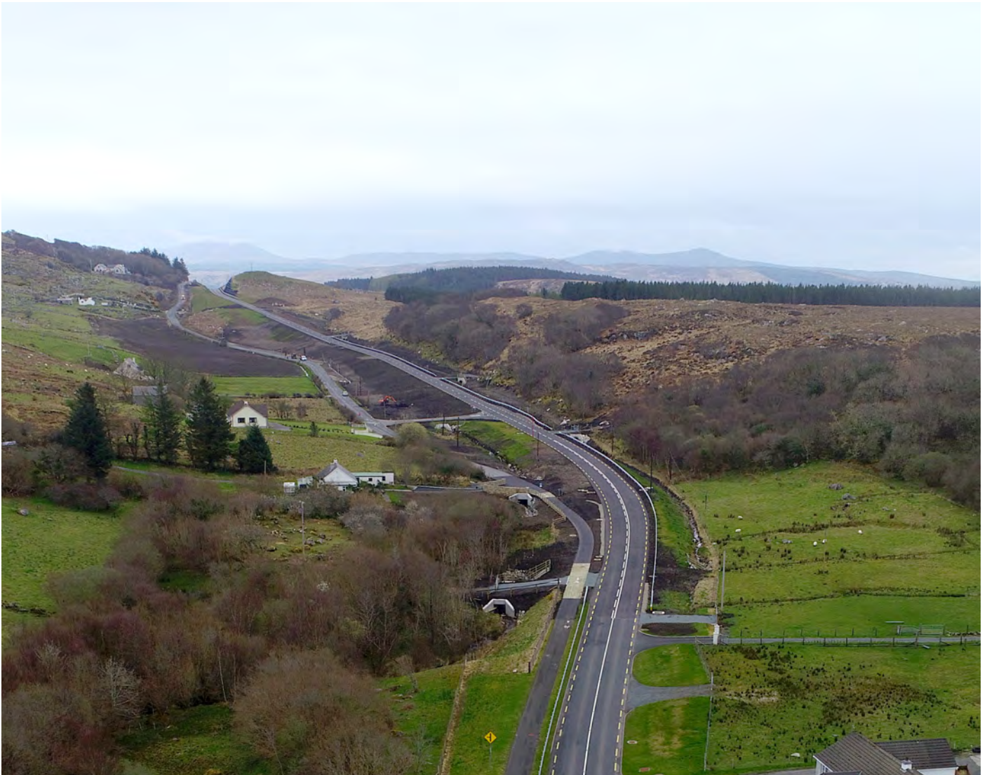
The northern end of N56 Letterilly to Kilraine Phase 1 project. A separate cycle track connects to the old road, passing the attenuation pond, realigned watercourse and culvert crossings for landowners accesses.
