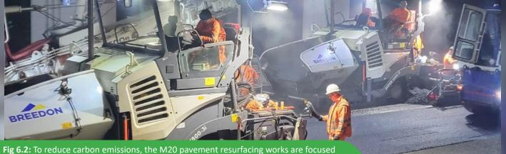
**Fig 6.2:** To reduce carbon emissions, the M20 pavement resurfacing works are focused on the trafficked road section only and do not extend to the hard shoulder.
