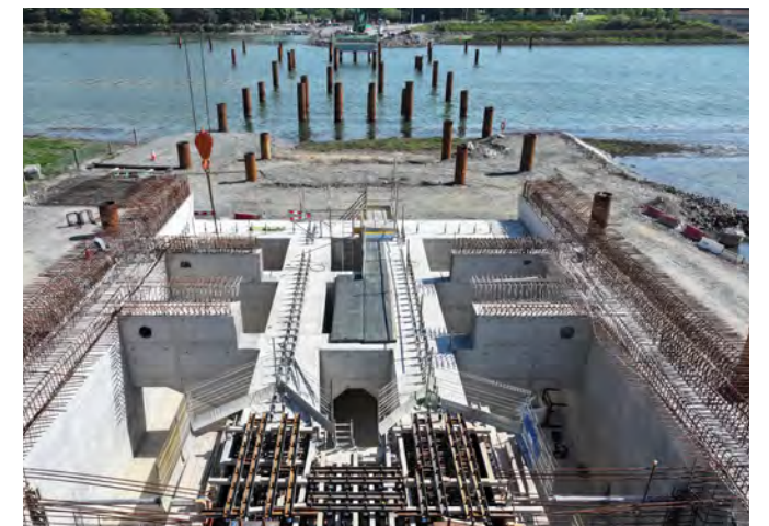
South Abutment – almost ready to receive the pylon & deck structural steelwork that is being fabricated off-site
