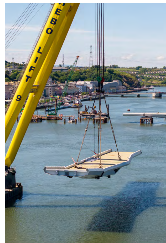
Sheerleg Crane lifting the sections into place.
