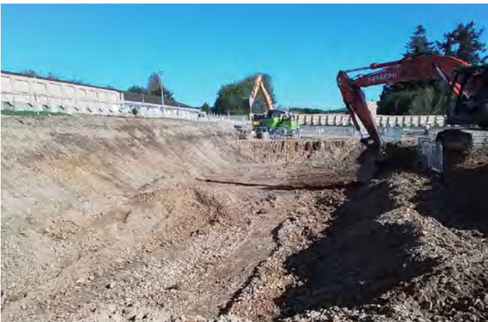
Excavation to formation level. Block 1 and Block2
