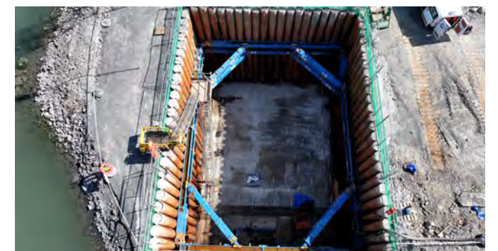
Bascule (North) Abutment cofferdam structure comprising an innovative Ruukki pile system – these piles will be integrated with the permanent works
