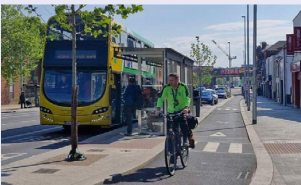
The scheme provided high quality, continuous, protected cycling facilities to meet existing and future demand.
