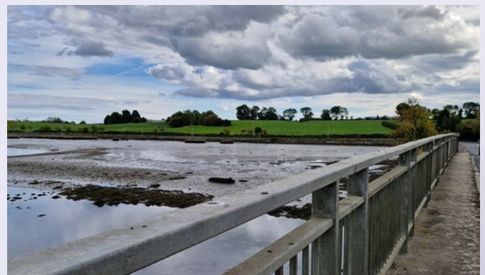
Shandon Island Bridge in Dungarvan, Co. Waterford.
