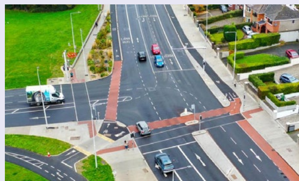
The scheme delivered improved pedestrian facilities by upgrading footpaths and installing additional pedestrian crossings along the route. Image courtesy of Dublin City Council.
