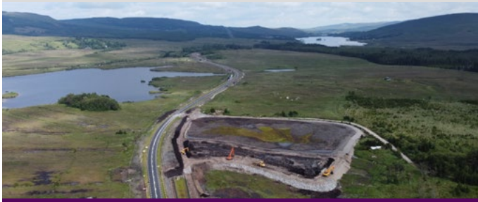
Peat deposition area constructed as part of N59 project near Maam Cross, Co. Galway.
