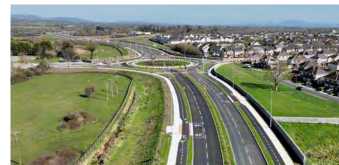
An aerial view of the link road between the Coonagh and Cratloe Roundabouts, which is located next to a residential area.
