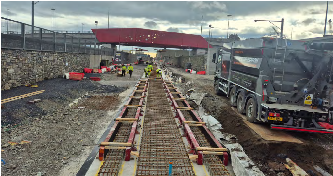
Construction of the Alexandra Road Project at Dublin Port.
