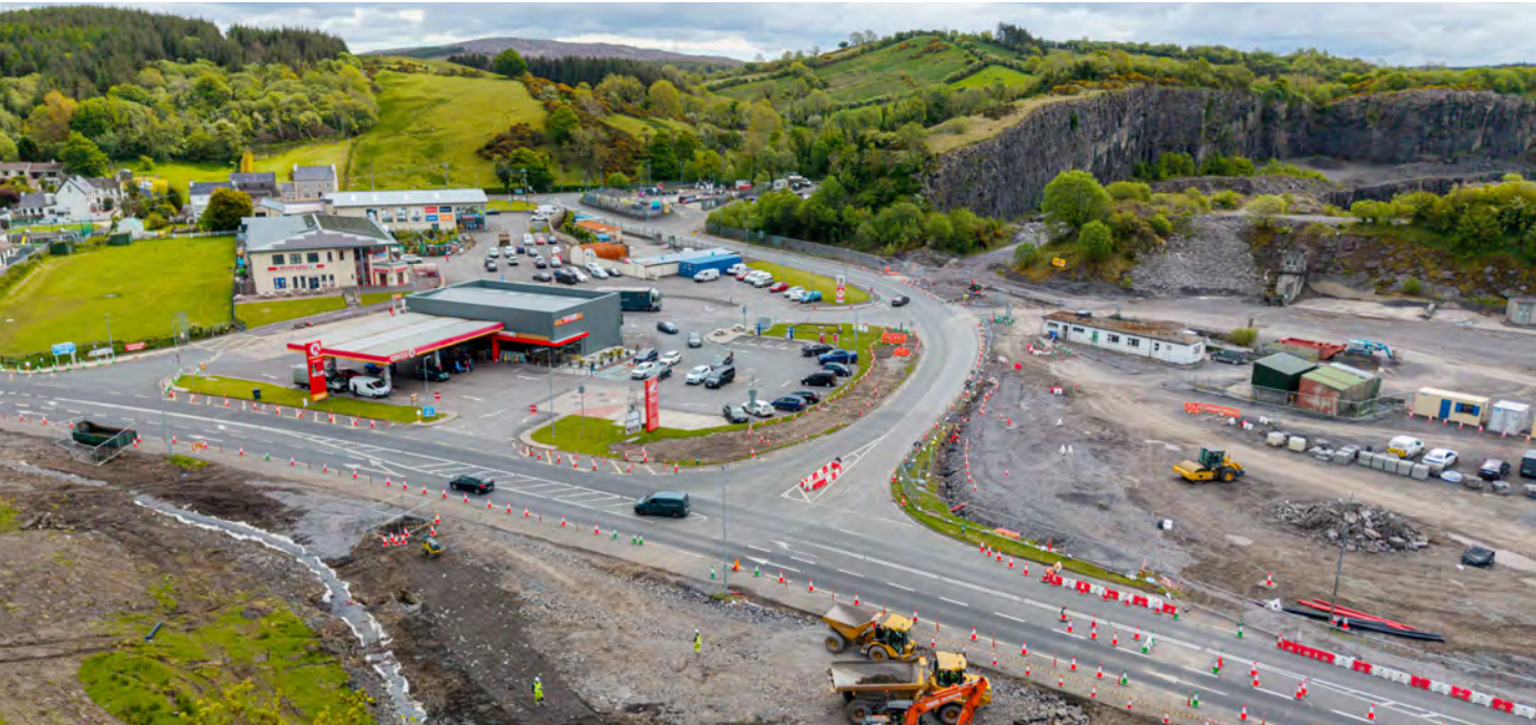
Laghey Roundabout on the N15 under construction.
