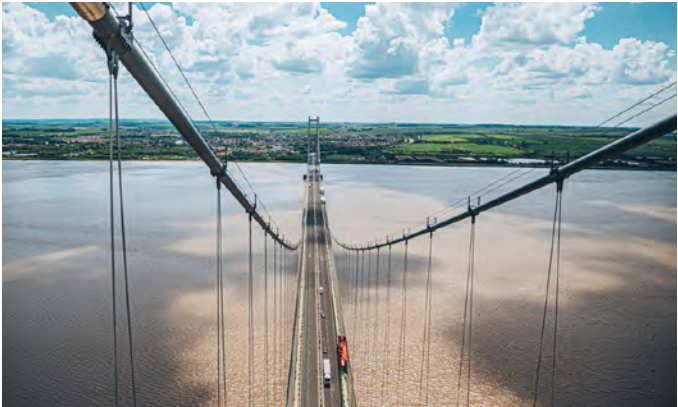
Looking south across the Humber Bridge from Hessle Tower during ROD’s 2022 inspection for the hidden defects study.
