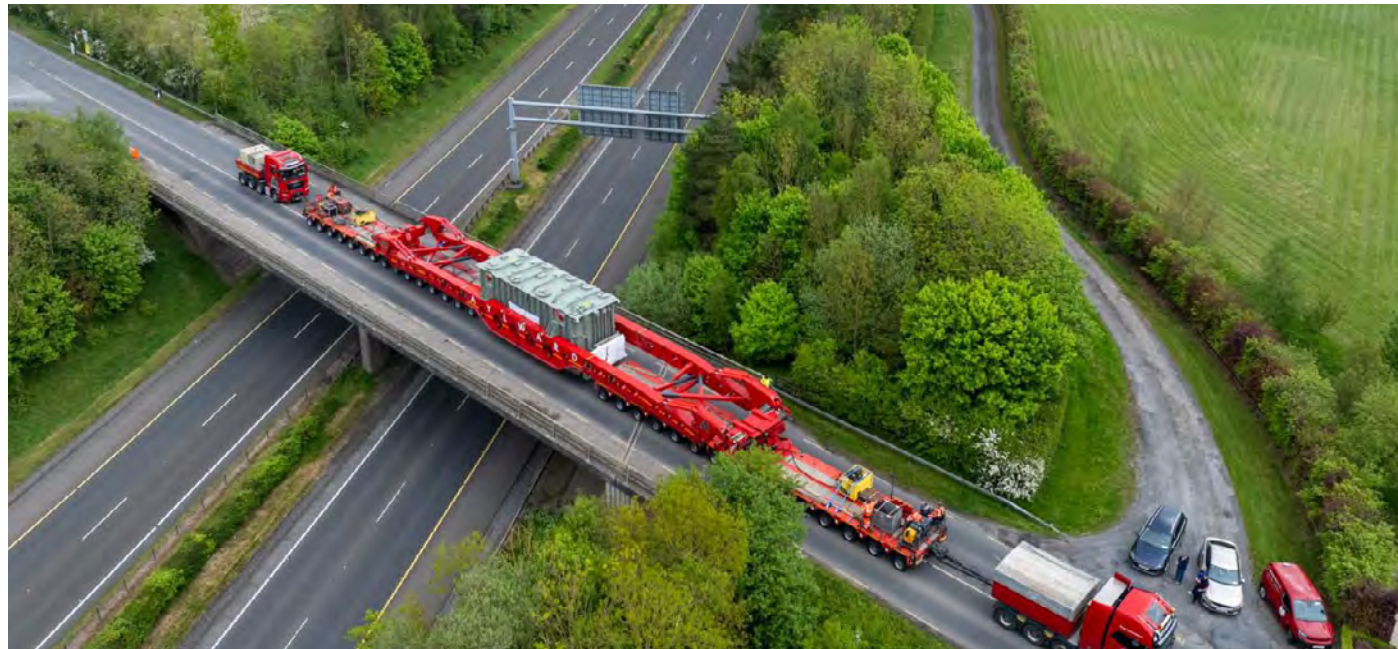
557 tonne Exceptional Abnormal Load crossing the M7.
