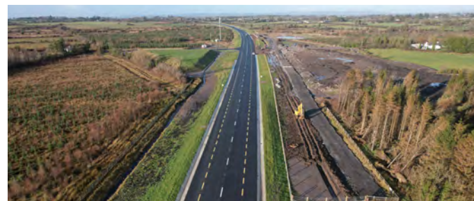
The first section of N5 road (near Frenchpark) being finalised for opening to traffic.
